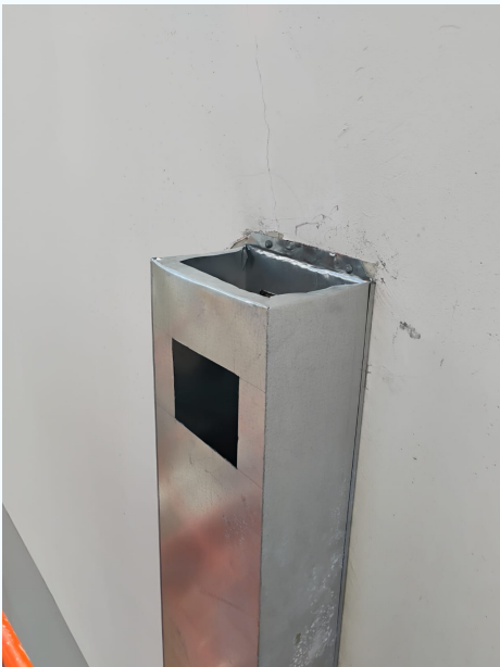
Downspout Installation
